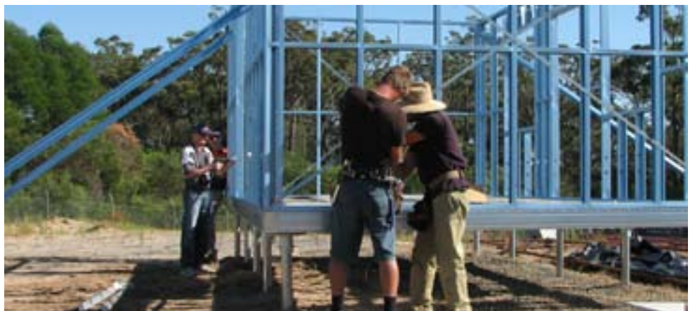
Wall frames being erected
